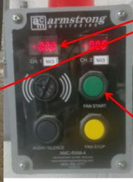
Detector displays (concentration in PPM). Systems may be equipped with multiple sensors (channels)
